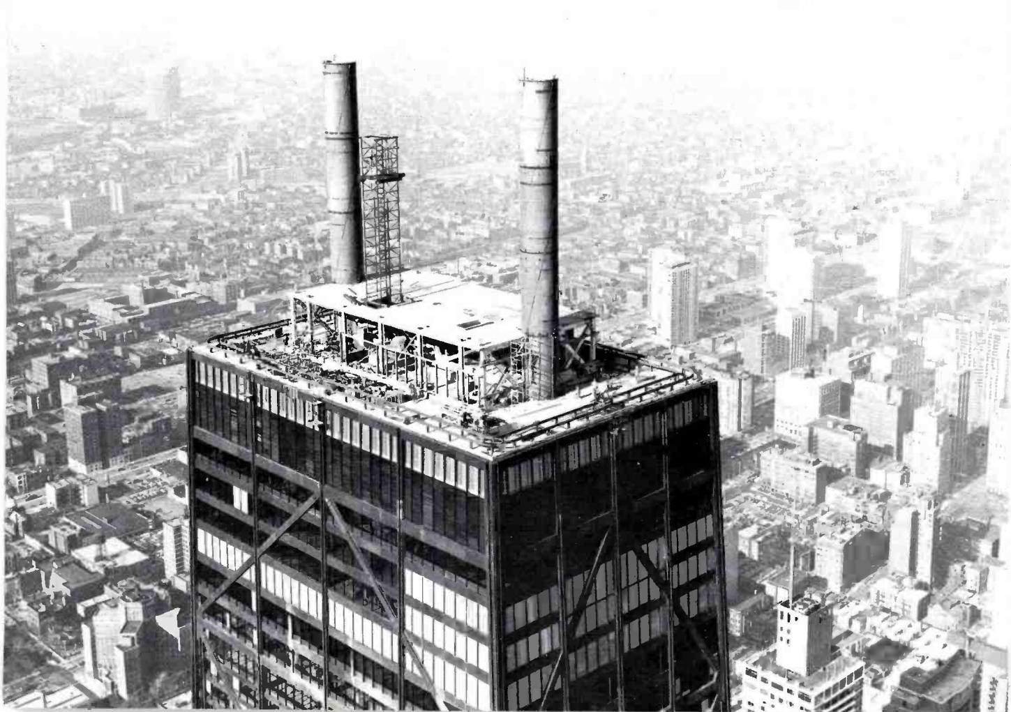
FIG. 3 Topside view of 100-story John Hancock Center as it appears from the air. The twin, 100-foot steel bases for the TV towers stand out in this helicopter view of construction in December 1968. The view is to the Northwest.
